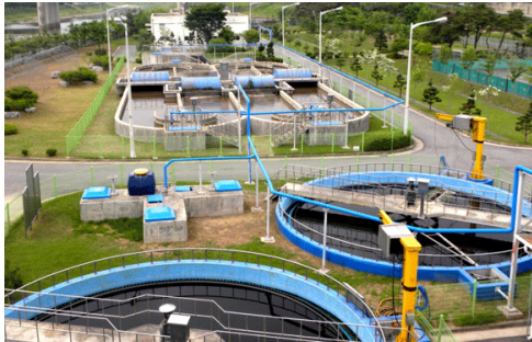
Fig. 4. Sejong City Public Sewage Treatment Facility
