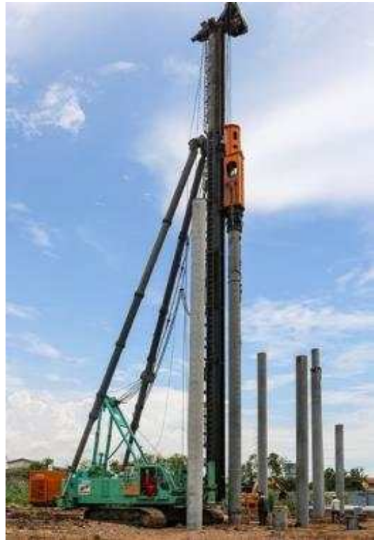
Fig. 8. General pile driving equipment
