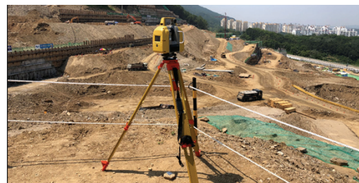
Fig. 3 3D laser scanner construction site application example (domestic)
