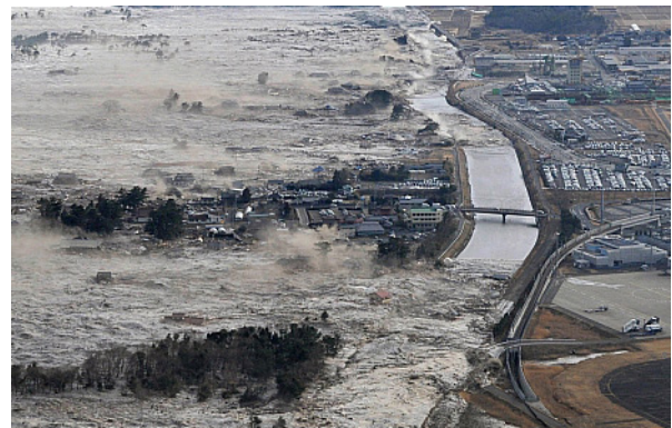
Fig. 4. Damage from the Tohoku earthquake
