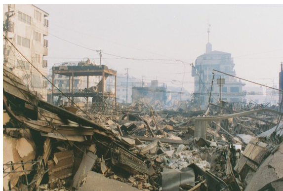
Fig. 1. Damage from the Kobe earthquake
