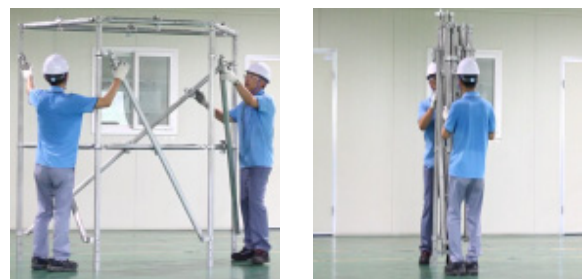
Unfolding Folding [Figure 2] Trapezoidal foldable scaffolding
