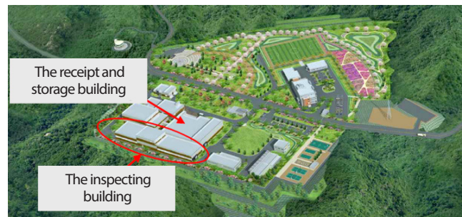
Fig. 1. Air view of the radioactive waste inspecting building.
