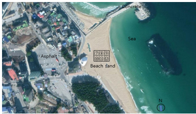
Fig. 3 Beach sand collection point for real data (Sokcho Beach)
