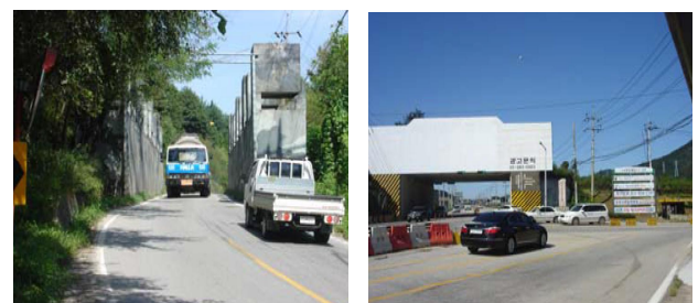
(a) Road bottleneck (b) Safety accidents caused by road structures
