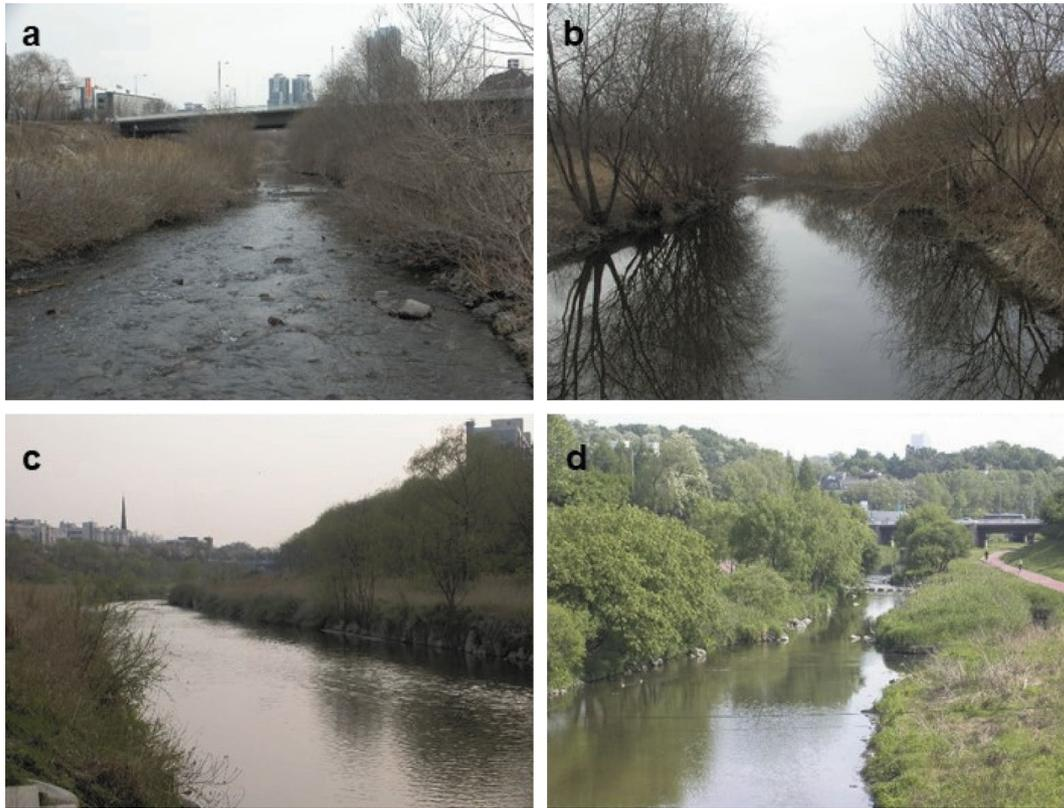
**Photo 1.** A feature of the restored Yangjae stream. The stream is composed of the double step sections and the slope of the section is steep (a). The introduction of vegetation does not reflect the flood regime, and thereby tree willow are introduced closer to the waterway than herbaceous reeds (b). On the waterfront, cobbles are piled up with steep slopes and trails for recreation are constructed (c), and thus reduce the naturalness and the ecological connectivity (d).
