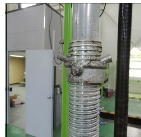
(c) Support pin destruction
