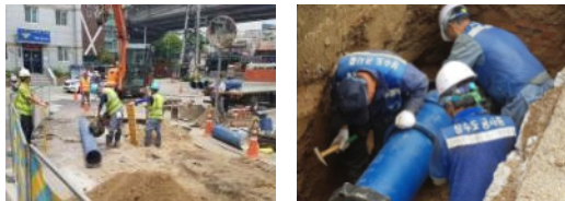
Fig. 5. Work status focused on plumbers
