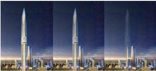
Fig. 6. Tower Infinity, which will be built in Incheon Cheongna International City, is the world's first transparent skyscraper. When the images of the surrounding landscape taken by the high-resolution cameras installed on the six sides of the tower are processed in real time and shown through the LED facade system installed on the outer wall of the building, an illusion in which the building disappears is created[16-17].
