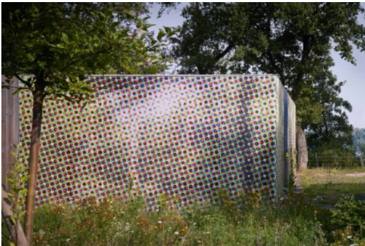
Fig. 5. The CMYK House is a housing project located near Moers, Germany. The outer wall wrapped in color halftones is a mixture of cyan, magenta, yellow, and black dots when viewed up close, but it is intended to make it difficult to recognize the shape of the pavilion mixed in a dense forest when viewed from the far away lakeside[15].
