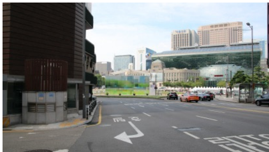
Fig. 9. A complete view of the installation seen from a distance of 100m.
