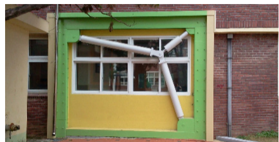
(Fig. 1) Seismic system using smart frame (Britec)
