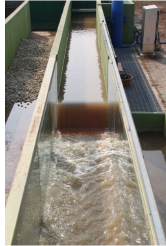
Fig. 3. Overflow at weir in channel.
