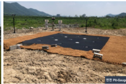
(c) Pit-Gauge Installation
