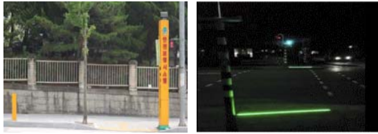
I-Safe lights system LED floor signal lights system
