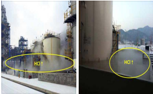
Fig. 2. Atmospheric dispersion of hydrochloric acid from the Dike[16].
