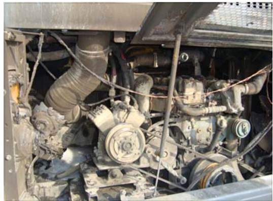
b) Acoustic absorbent installing part of engine room
