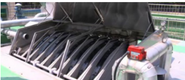
Fig. 2. Fiber disc-filter to treatment discharge water in A-WTP.
