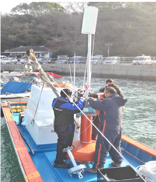
Fig. 10 Aids to navigation with radar reflector
