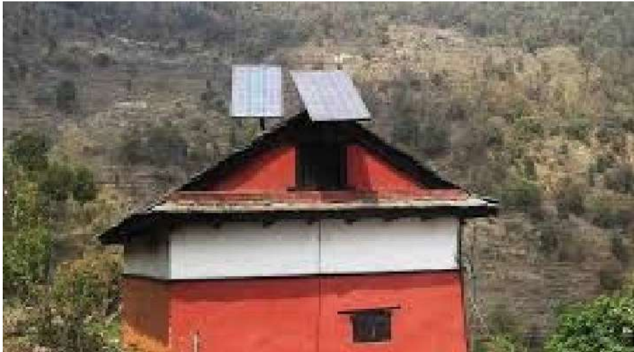
Figure 5. Solar PV systems installed in Chhelurng, ward no. 13, Tansen Municipality, Nepal
