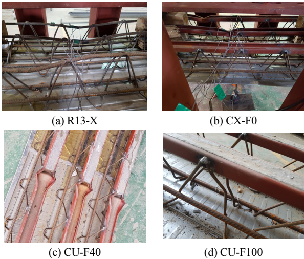
Fig. 6 Failure mode of specimen
