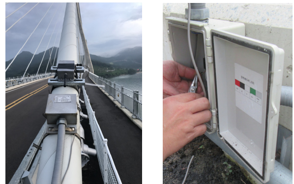
Fig. 2 Installation of LoRa sensor node and power
