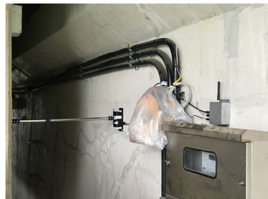
Fig. 3 Installation of LoRa sensor node for DAQ
