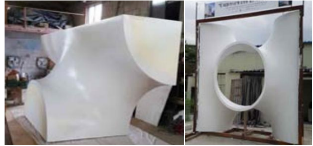
Figure 1. EPS form & mock-up for Hanabank remodeling work
