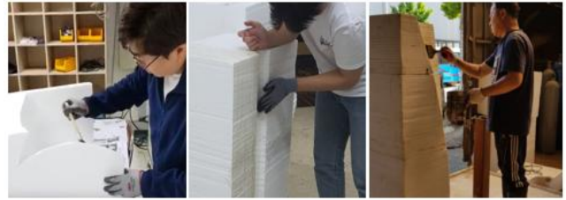
Figure 7. Spreading polyurea & taping & spreading form oil
