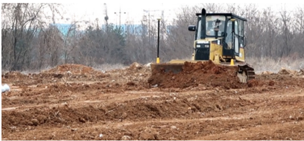
Fig. 5. Machine guidance dozer grading work
