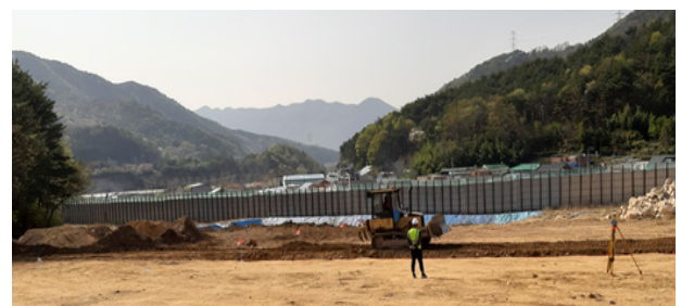
Fig. 3. General dozer grading work
