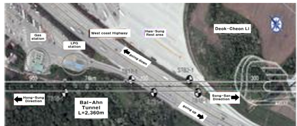
Fig. 5. 00 Low Depth Railway Tunnel Construction Site
