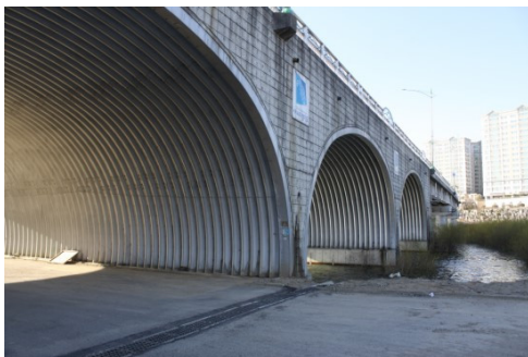
Fig. 1. An Example of Corrugated Steel Plate Bridge
