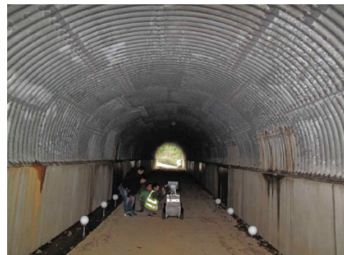
Fig. 9. Corrugated Steel Plate Culvert for Safety Assessment
