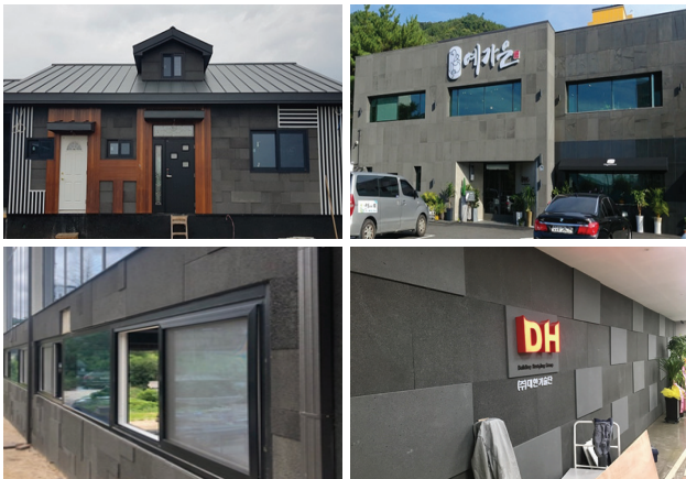
Fig. 1. Application of non-flammable mineral foam board
