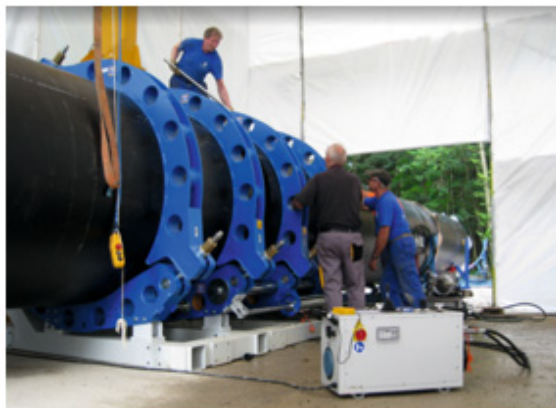
Figure 9. Butt fusion in a protective shelter (photo courtesy of +GF+, Switzerland).
