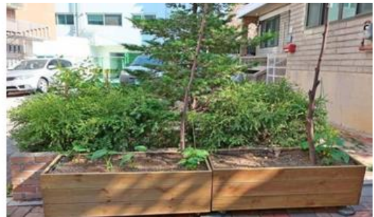
(b) rainwater harvesting tank
