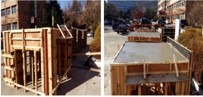
Figure 3. Form of specimen and concrete curing
