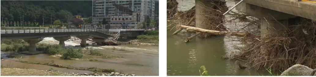
Fig. 1. Bridge collapse and deposition of driftwood around bridge piers (<https://news.kbs.co.kr/news/view.do?ncd=5001887>).
