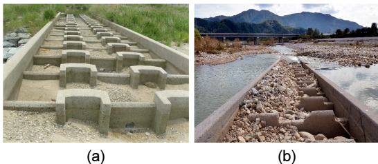
Fig. 1. Poorly constructed ice harbor-style fishway (a) Ice harbor-style fishway in Bulyeong Valley, Ulsin-gun, Gyeong-sangbuk-do, (b) Ice harbor-style fishway in Seongju-gun Daega river.
