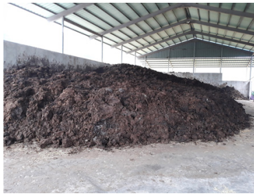
Stack type composting facility
