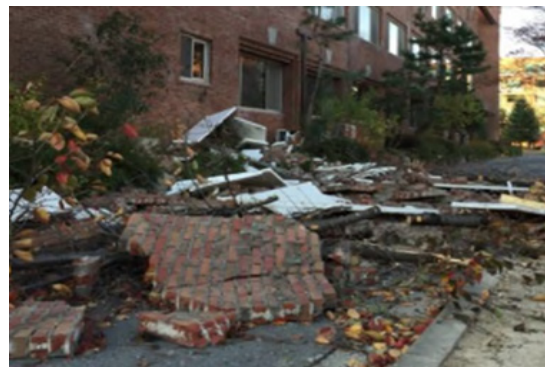
〈Fig. 1〉 Failure of the masonry walls
