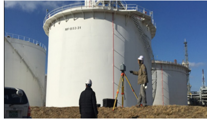
Fig. 2. Oil Storage tank
