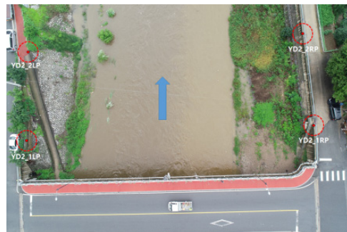
(b) Yeongdong-gun (Youngdong 2nd Bridge)
