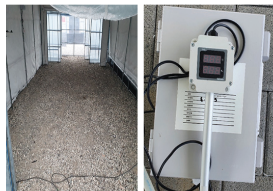
Fig. 3 Green house with temperature/humidity sensor node and Aerogel installed
