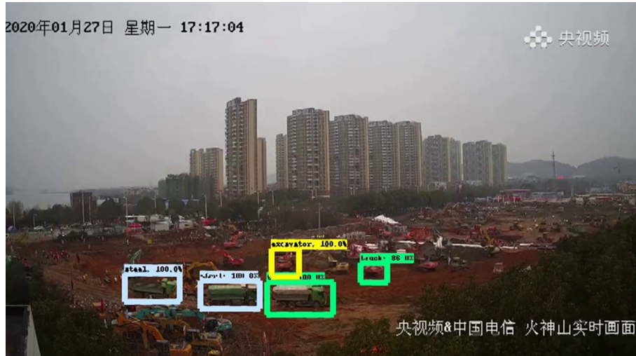
Figure 8. Detection Result in Huoshenshan Hospital.
