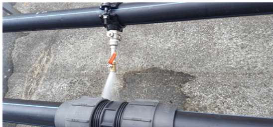
Fig. 8 Valve installed in PE piping
