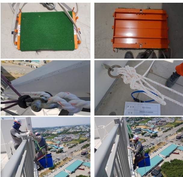
Fig. 3. Scaffolding Work Progress
