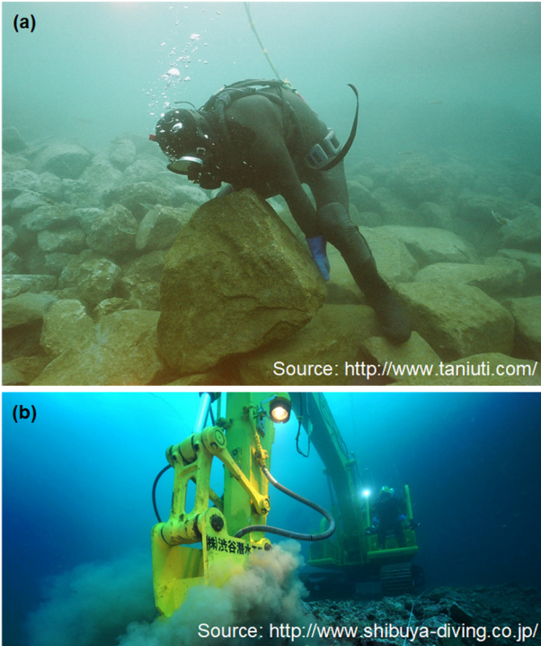
Fig. 1. Underwater operations by diver and heavy equipment in hyperbaric environment.
