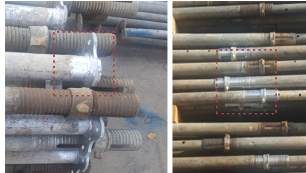
Fig. 2. Pipe welding and replacement of support structures.
