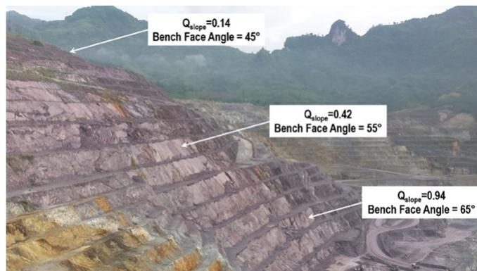
Fig. 1. Changing geologic structure orientations (steepening of bedding planes down slope) help to explain the appropriately steepened bench face angles in a large opencast mine setting, Laos.(after Barton & Bar, 2015)
