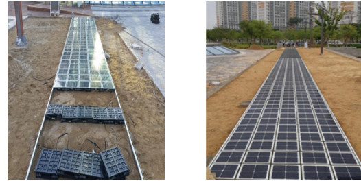
Fig. 10. Road solar module installation process.
