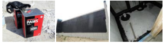
Fig. 7. Asphalt Waterproof Applying Area
