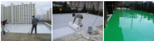
Fig. 6. Liquid-applied membrane waterproofing construction Method
