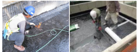
Fig. 8. Sheet waterproofing construction Method
