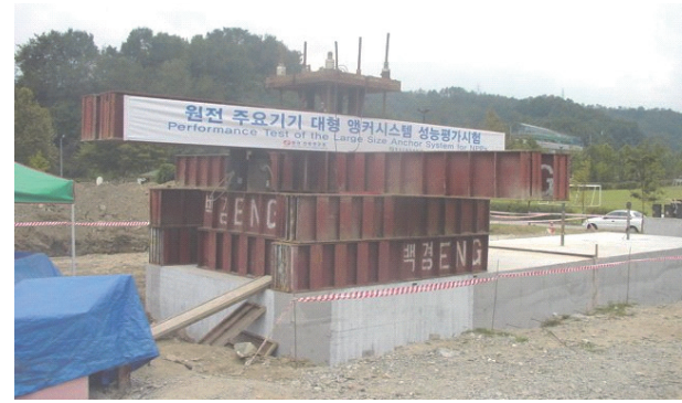
Fig. 3. Photograph of actual tensile test setup.
