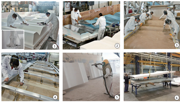
Figure 6. Precast FRP module development process (Source: Kreysler & Associates, Enclos Company)
