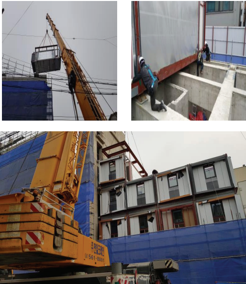
Fig. 1 Field installation of modular
