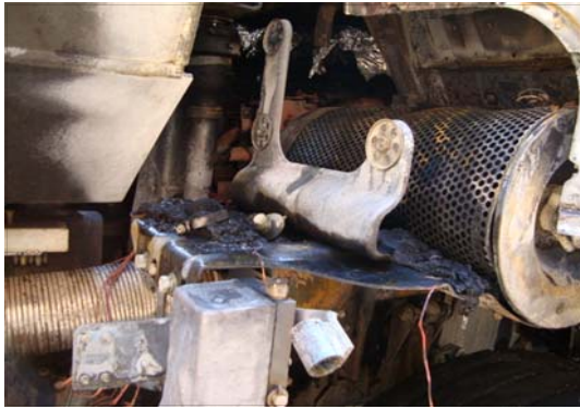
Fig. 2. Fire example by wire short causing coolant leakage on air cleaner part.
